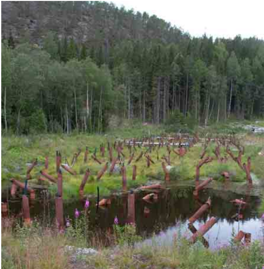
Figure 5.1 The frozen construction site at the Bothnia Line in July, 2007, approximately five years after the cooling machine was turned off. Chainage 13+615 in the foreground and chainage 13+520.5 in the background near the mountain, Stranneberget. The visible parts of the freeze pipes have been cut off at the present ground surface level and will be covered by a soil layer and joined with the adjacent ground surface
