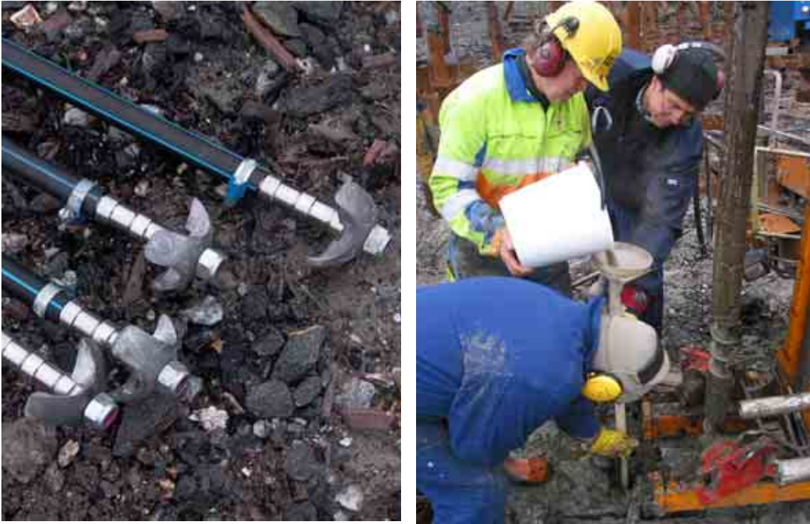
Figure 5.11 Installation of ground level gauges. Illustration to the left; ground level gauges with protection casing (four). Illustration to the right; sealing of the mounted ground level gauges with sand
