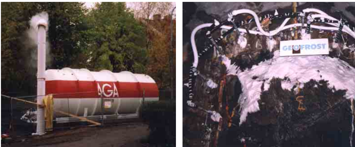
Figure 2.10 Cooling by direct expansion at the project Älvsjö storm water tunnel. The picture on the left-hand side shows the interim storage tank for liquid nitrogen. The picture on the right-hand side shows the freeze pipes organized at the tunnel arch. Photo Lasse Wilsson, Skanska
