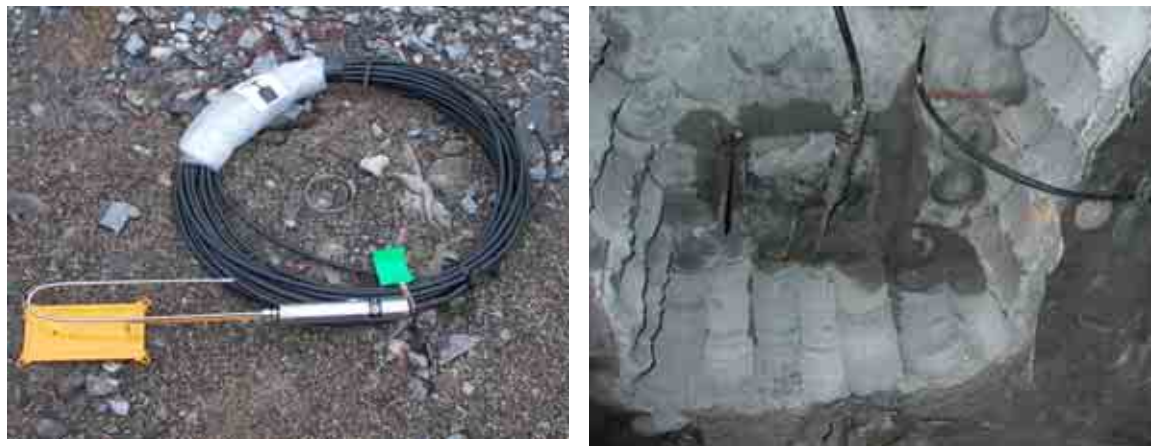
Figure 5.8 Installations in the tunnel at the Bothnia Line, figure of the left-hand side, soil pressure cell to be installed. Figure of the right-hand side, soil pressure cell installed above the insulation behind 0.25 m shotcrete
