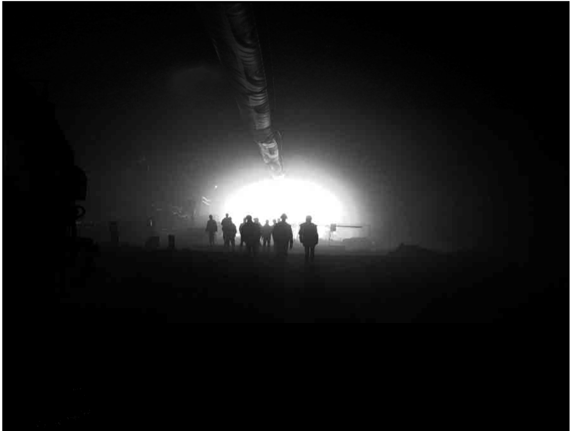
The Håggvik tunnel in the spring of 2005 (Stockholm)
