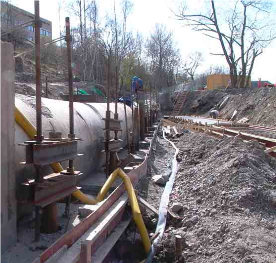
Figure 1.1 Artificial ground freezing as an aid in tunnelling in the central of Stockholm, origin a thaw settlement of a 1.2 m in diameter shallow concrete sewer above the stabilized tunnel. Rescue operations of the settled sewer failed (on the left-hand side) and a brand new bypass sewer was built (on the right)
