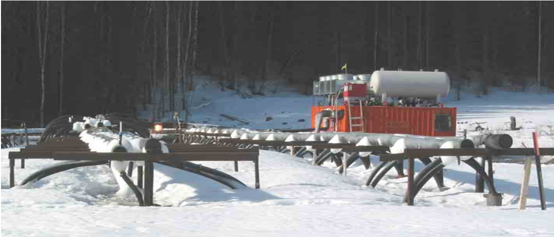
Figure 1.2 Artificial ground freezing at one part of the Bothnia Line. In front of the mountain, Stranneberget, on the left-hand side, the brine supply systems for the installed freeze pipes in the ground. On the right-hand side, the cooling device, i.e. the storeroom of the cooling machinery
